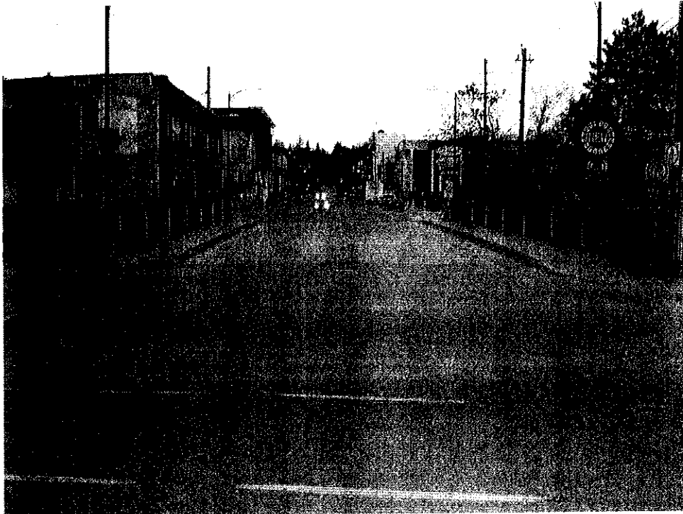
Photo 1 (IMG-1034)– View of the structure looking East.
