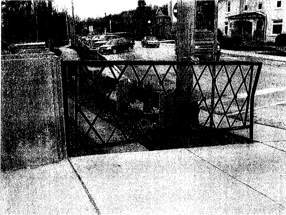
Photo 9 (IMG-1048) – South west approach guide rail is permanently deformed and sections are missing.
