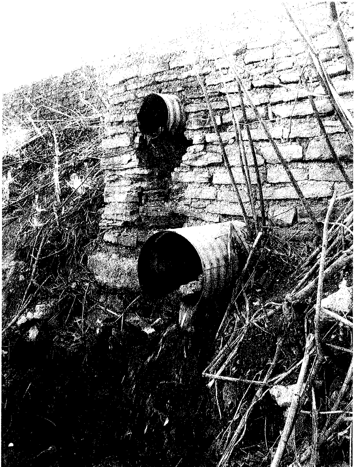
Photo 19 (IMG-4757) – Steel culverts in south west retaining wall. Note both bottoms are badly corroded. The water is causing very severe disintegration of the retaining wall.
